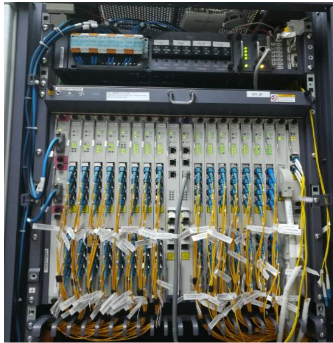
Figura 4.4 OLT Huawei
